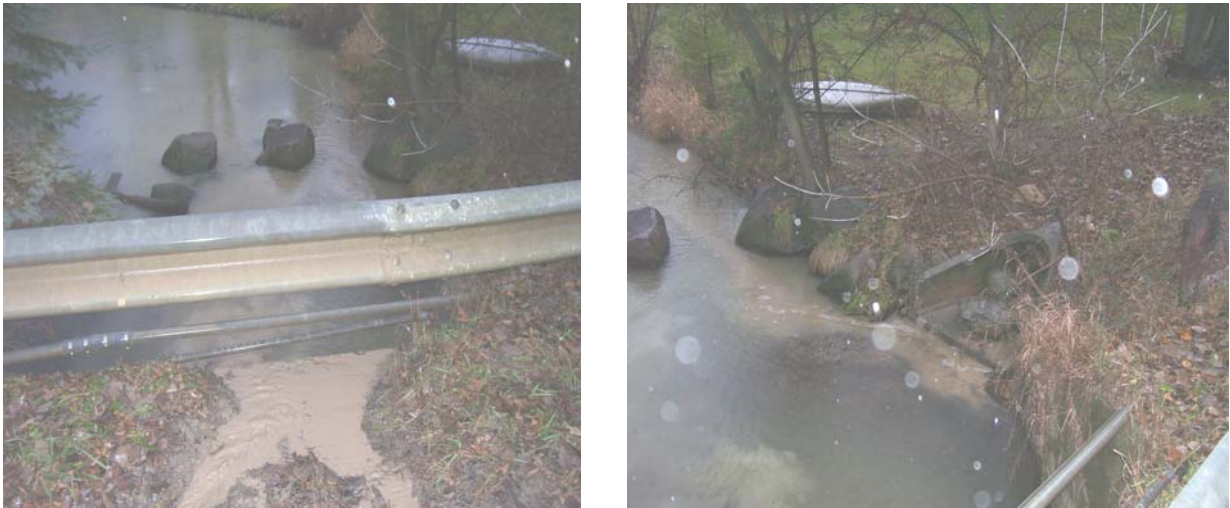
Figure 2: Runoff entering Mann Creek from Pleasant Valley Road and from the drainage system
